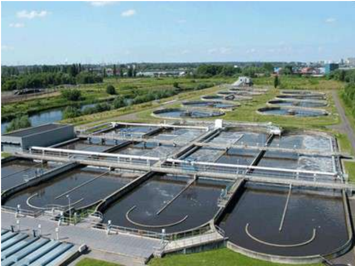
Planta de tratamiento de aguas residuales http://making-biodiesel-books.com/algae-bioproducts/algae-wastewater-treatment/
